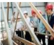
Build a big building
